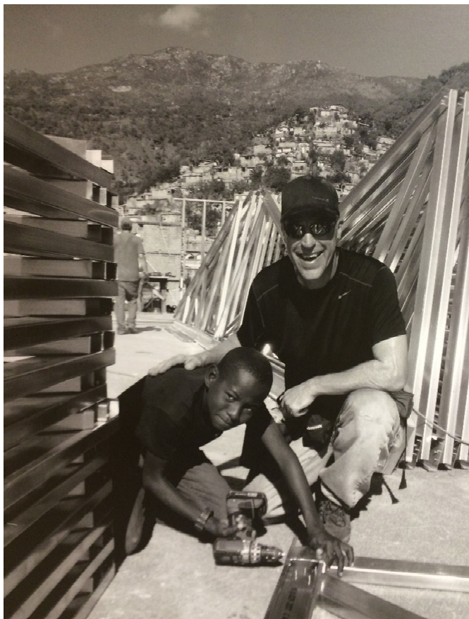
Wyatt helped build light-gauge metal trusses on-site in Cap Haitien, Haiti.
